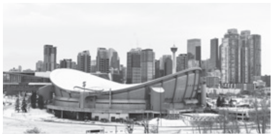
Construction of the Saddledome, the home of the Flames, began before the Olympics were awarded in 1981, adding credibility to Calgary's bid for the games. With its iconic hyperbolic paraboloid roof form, it was the principal venue for ice hockey and figure skating competitions. The building is near the end of its safe and useful lifespan and will likely be replaced with a new arena and concert venue in the near future.
